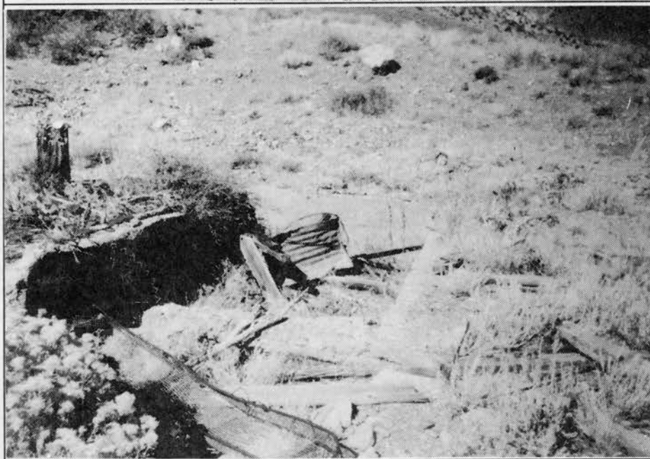
Rubble and concrete foundation
