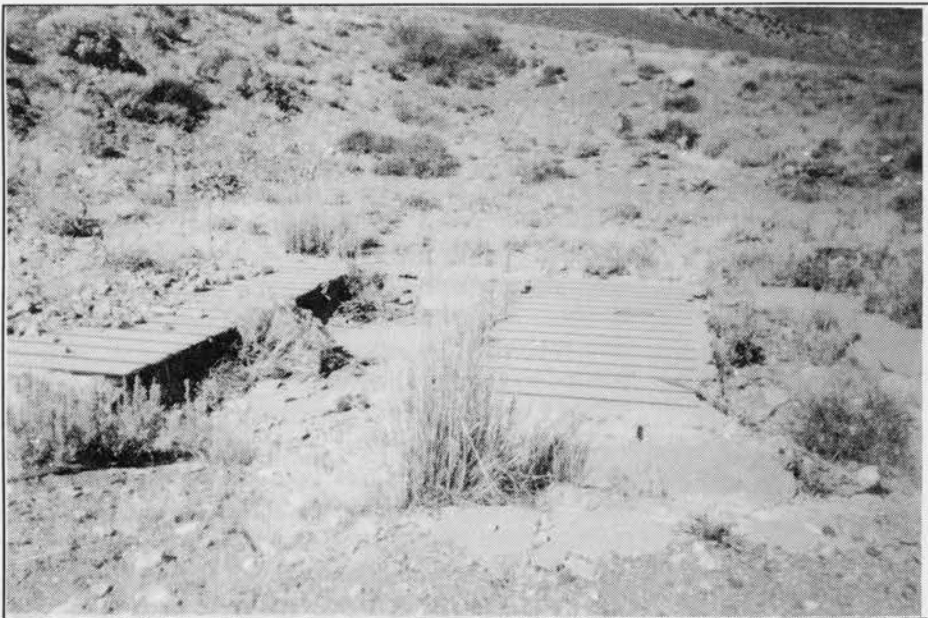
Foundation of the Jordan Power House
